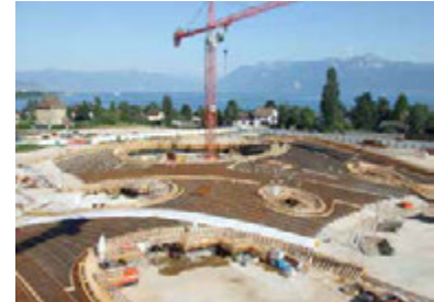
FIG. 5.4.4 construction of the slab for larger hill in 2008 (Grohmann 2008)
