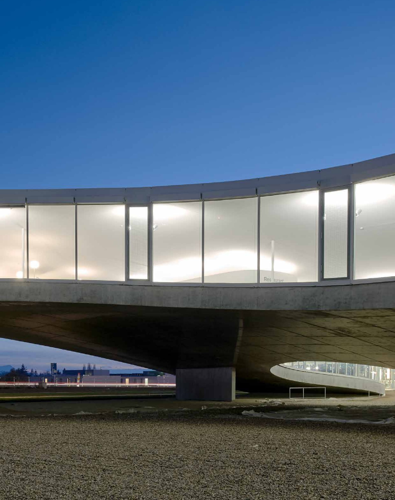
FIG. 5.0 Rolex Learning Centre at EPFL, Lausanne SANAA 2004-2010 (Photo: Ariel Huber)
