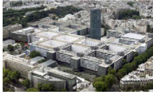
FIG. 4.4.2 Jussieu Campus asbestos removal (Reuters 2011)
