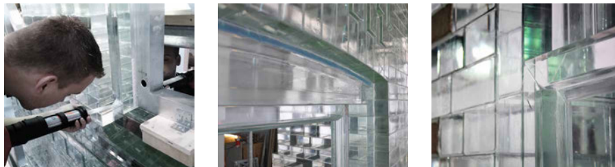
FIG. 6.23 Left: The simultaneous application of the polymer from both sides. Centre and right: The final result of the bonded glass frames.
