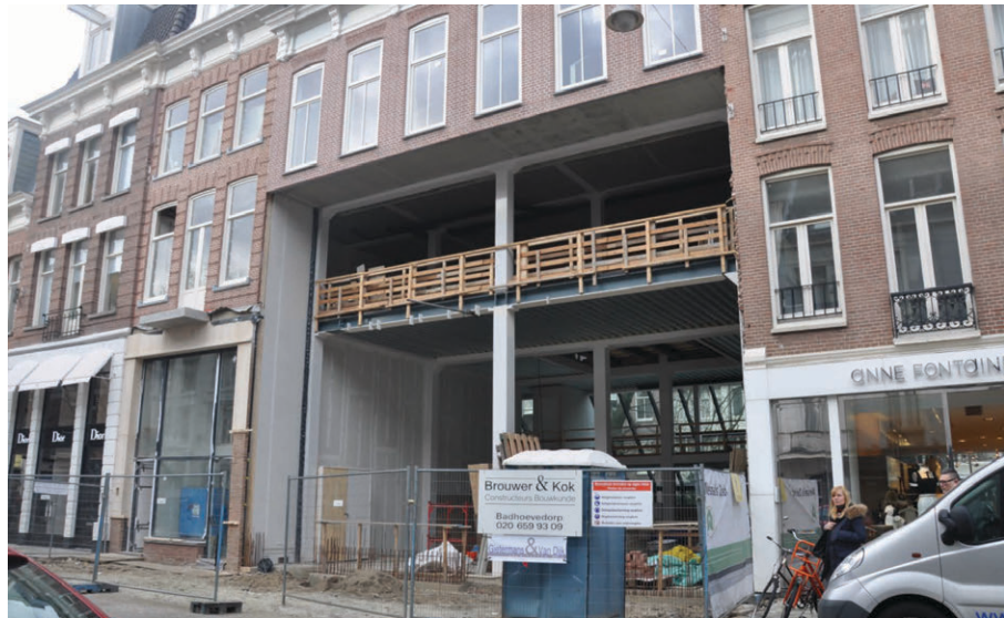
FIG. 6.8 The masonry wall was already constructed prior to the glass elevation.
