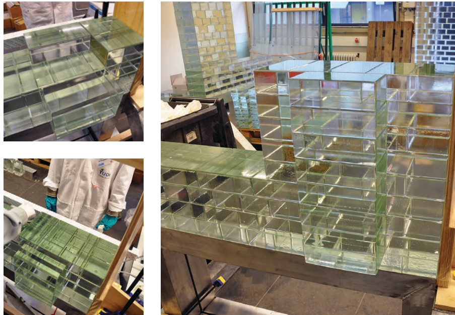
FIG. 5.8 The final (4th) wall mock-up which includes the buttress's construction by interlocking glass blocks
