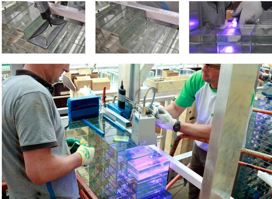
FIG. 4.18 Bonding and curing of the adhesive at the Crystal Houses façade.
