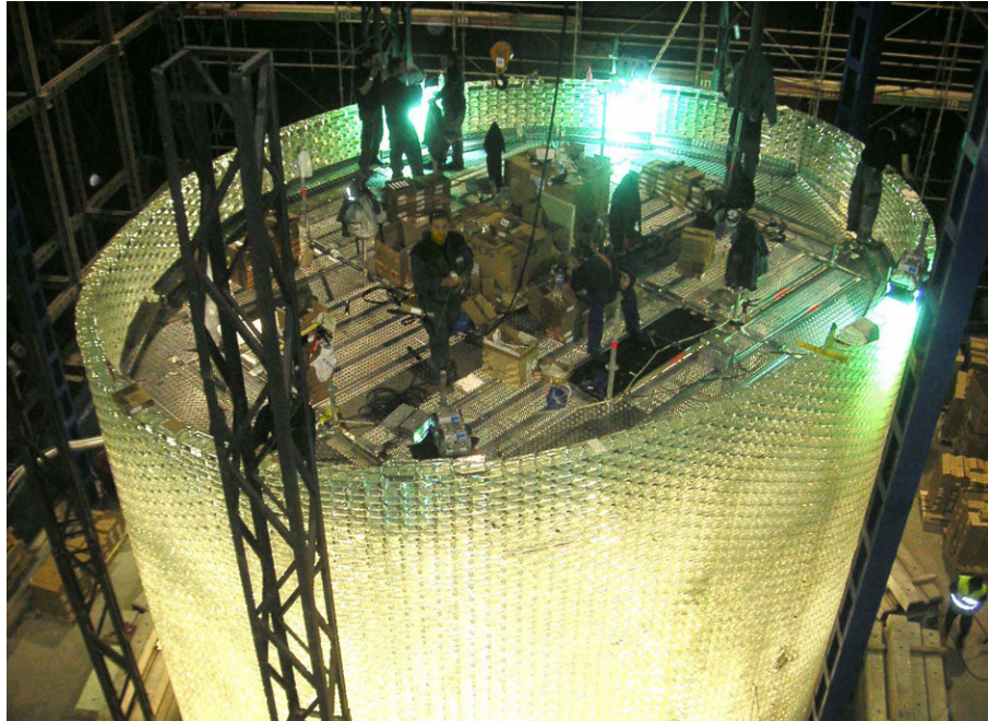
FIG. 4.12 Construction of the Atocha Memorial. Source: Bellapart, SAU.
