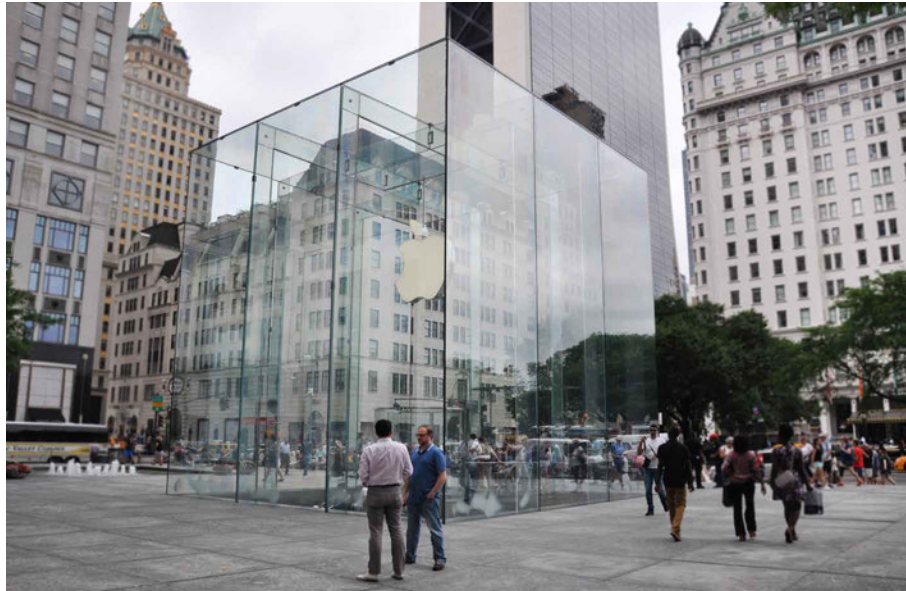
FIG. 1.1 The Apple Store in New York by EOC Engineers
