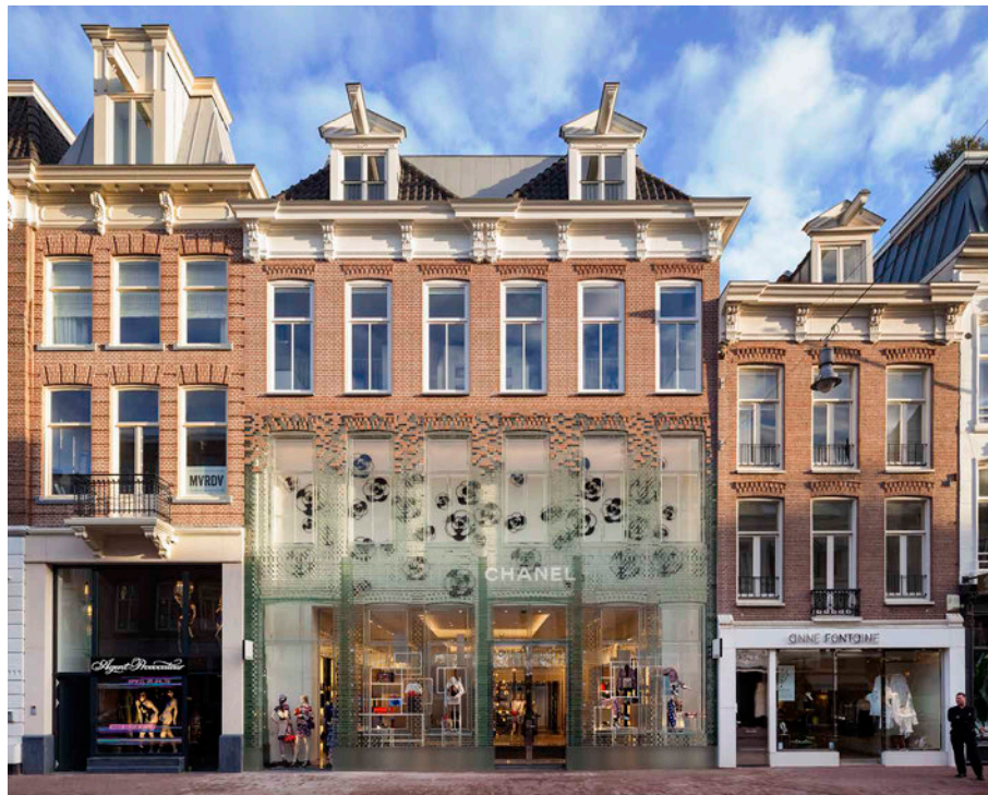
FIG. 1.2 The Crystal Houses façade in Amsterdam by MVRDV Architects , made of adhesively bonded glass blocks. Source: Daria Scagliola and Stijn Brakke .
