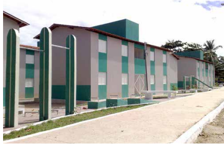
FIG. 5.9 Pictures show the housing project Vila S. Pedro in 2009 (after delivery). Source: Agência Alagoas, 2010.
