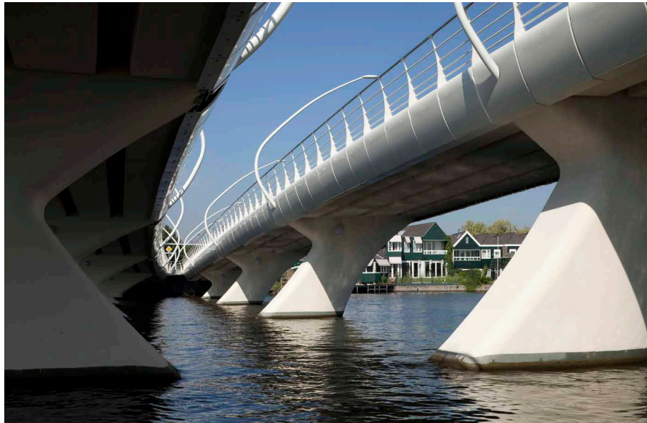
FIGURE 2.10 Pedestrians and cyclists have a bridge of their own. A void separates them from motorised traffic. Royal HaskoningDHV, Joris Smits et al. (2013). Photo by Luuk Kramer 2009.
