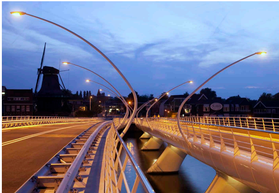
FIGURE 2.14 Light masts define the space and viewing directions. They emerge from the void in order not to obstruct the outward view. Royal HaskoningDHV, Joris Smits et al. (2013). Photo by Luuk Kramer 2009.
