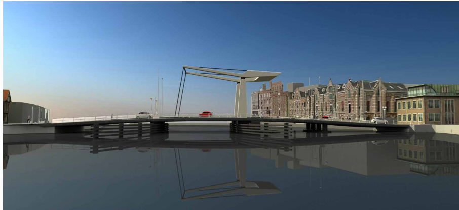
FIGURE 2.8 The Zaan Bridge in Wormer is of the traditional drawbridge typology. Approach spans and drawbridge form two different entities. Royal HaskoningDHV, Joris Smits et al. (2015).
