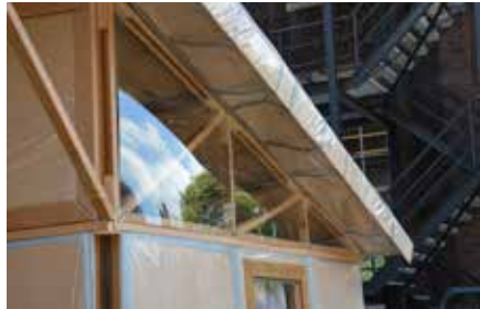
FIGURE 7.42 Roof structure made out of U-shapes
