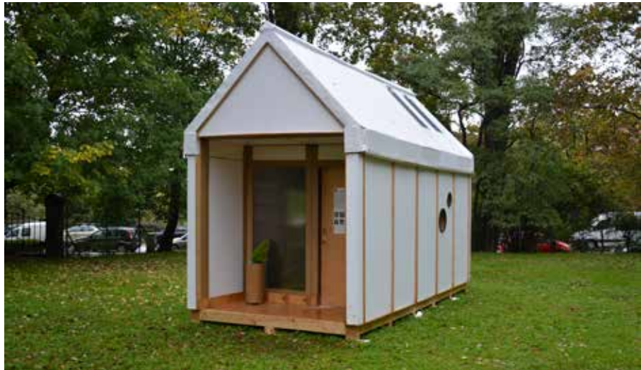
FIGURE 7.69 the House of Cards on campus of Faculty of Architecture, Wroclaw University of Science and Technology
