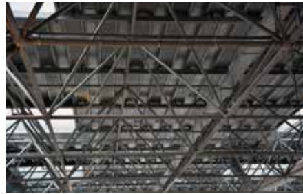
FIGURE 4.93 Space frame structure of the south-facing hall, Faculty of Architecture TU Delft, 2017
