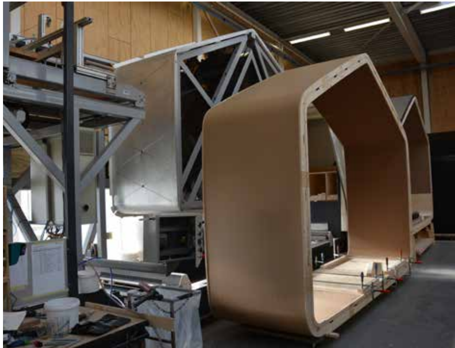
FIGURE 4.110 Wikkel House segments taken off the mould at Fiction Factory, Amsterdam, 2016
