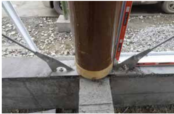
FIGURE 4.106 Foundations of Miao Miao Paper Nursery School, 2013
