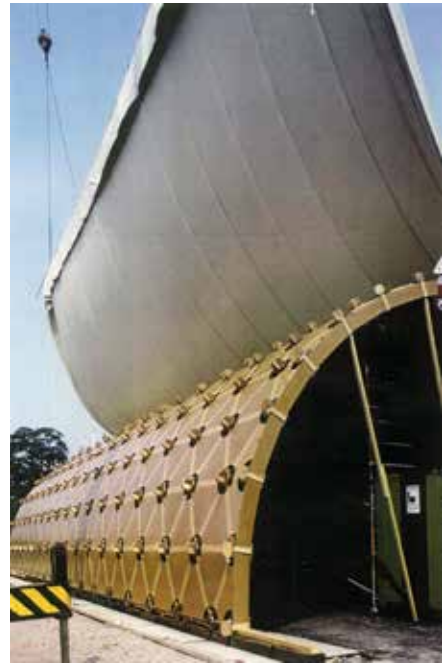
FIGURE 4.25 Watertight membrane covering the cardboard structure with a separate canvas membrane from the top downwards, 1992
