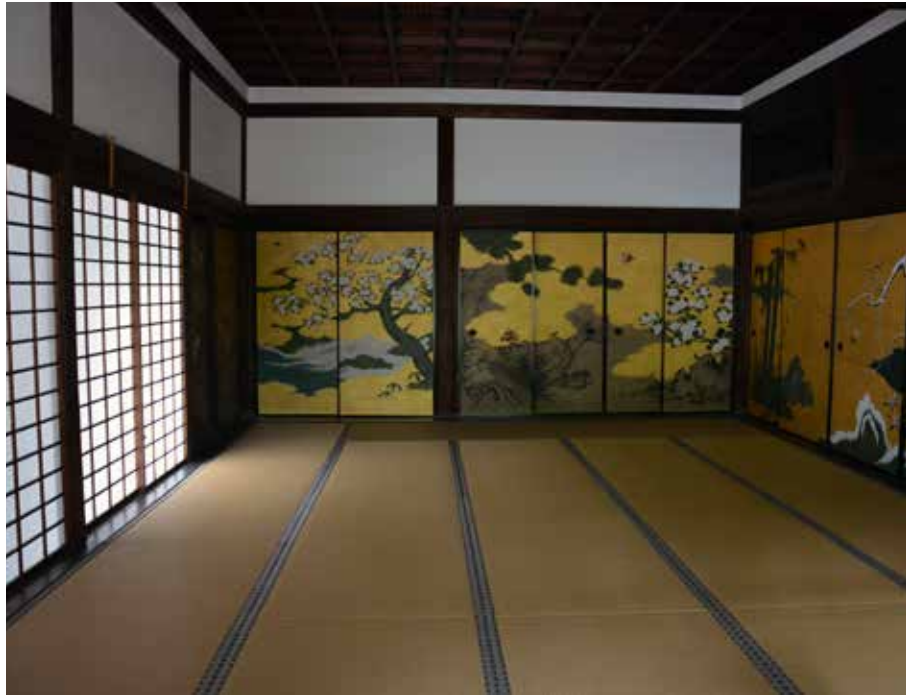
FIGURE 4.1 Shoji (translucent paper screens) and fusuma (sliding panels) in Nazen-ji Temple, built in Kyoto, Japan, in the thirteenth century AD, 2013
