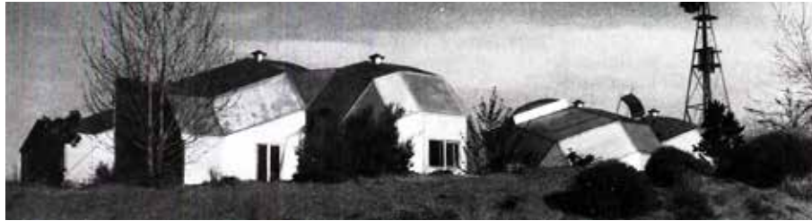
FIGURE 4.13 Baer Zome house, Corrales, New Mexico, 1971
