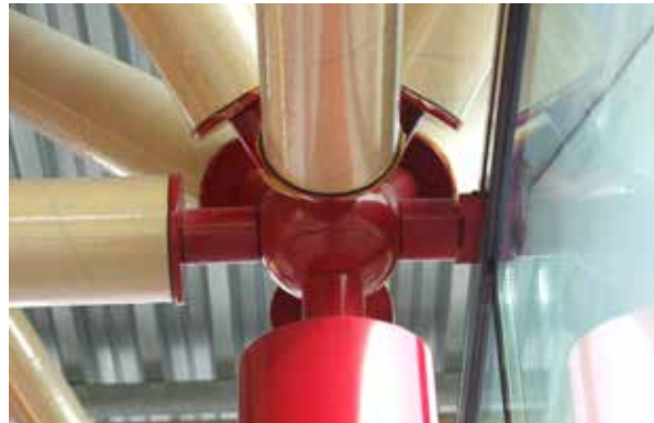
FIGURE 4.89 Ring Pass Field Hockey Club, Tuball – connection between paper tubes and steel column, 2012
