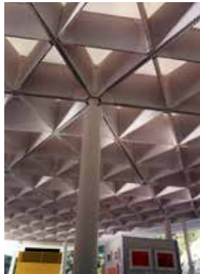
FIGURE 4.53 Nemunoki Children's Art Museum roof structure and construction, 1999
