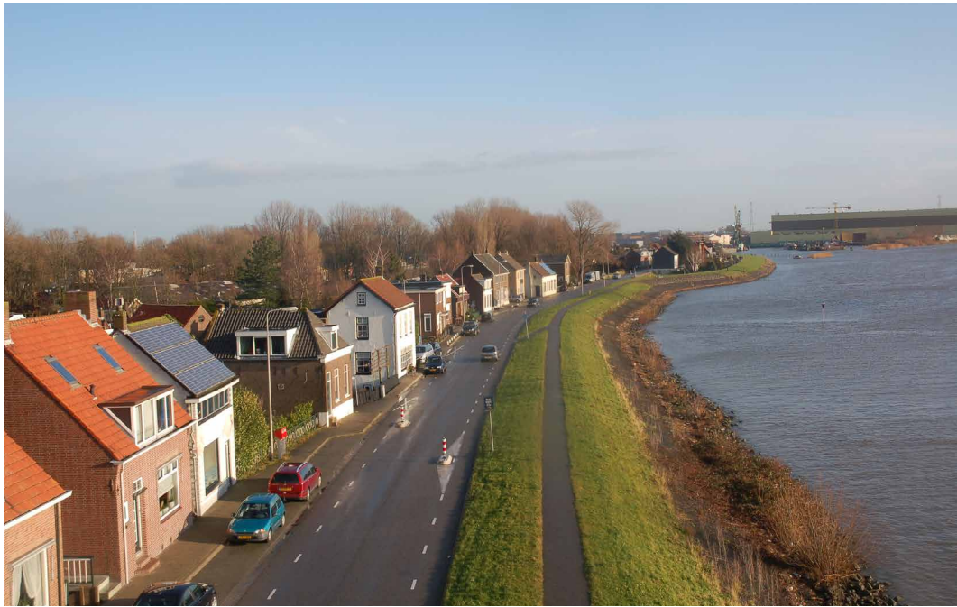
FIGURE 5.5 Photo of the Sliedrecht levee along the Merwede, incidental built constructions and trees on the riverside have been removed for dike reinforcements
