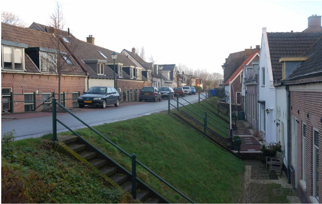
FIGURE 5.7 Photo of a previous levee elevation on a two-sided built levee along the river Lek near Everdingen
