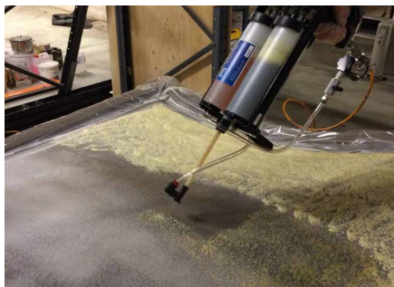
FIGURE 6.16 Applying the HDPU
