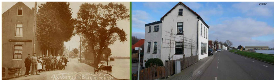
FIGURE 8.7 On the left, a historic photo of the Sliedrecht dike, showing the historical presence of trees and buildings in the unbanked area along the river. The trees were removed to accommodate for dike reinforcements, changing the spatial characteristic of the dike ribbon. The picture on the right shows the current situation. Photos: Sliedrecht historic society ( http://www.historie-sliedrecht.nl ).
