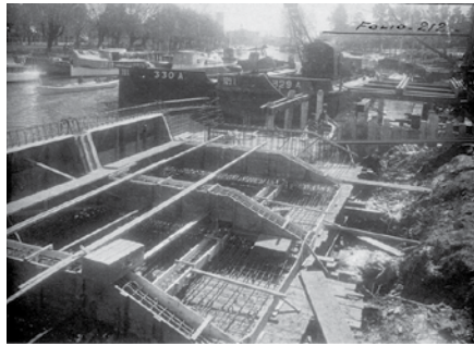
FIGURE 4.32 Dike construction in the port of Tigre in 1934 (Histarmar, 2016).
