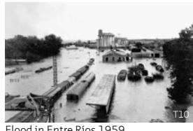
Flood in Entre Rios 1959
