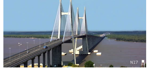
2003- Construction of Rosario-Victoria 4 Km-long Bridge (RN174) ▶
