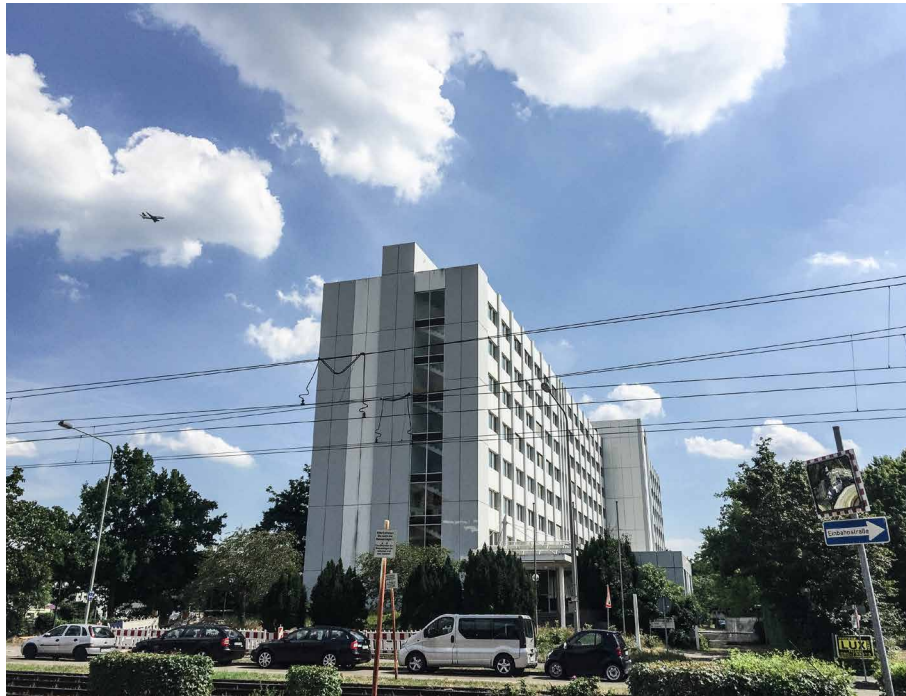
FIGURE 4.20 Lyoner Straße 54, Frankfurt, the abandoned office building on Lyoner Strasse 54, picture by the author.
