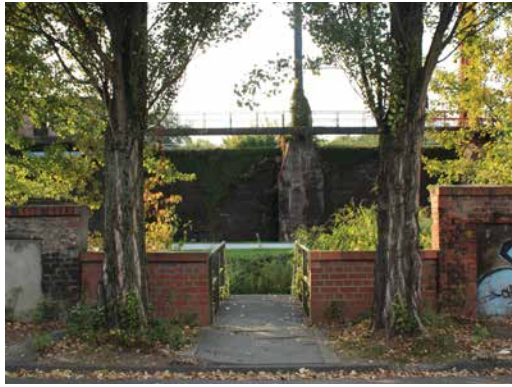
FIGURE 7.33 Belvedere platforms, Klarwasserkanal. (Photo: Author).
