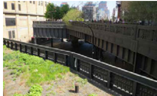
FIGURE 8.31 Northern Spur & 10 th Avenue Square. (Photo: Author).
