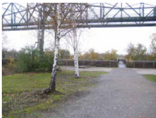
b Bunker roof entrance area. (Photo: Author).
