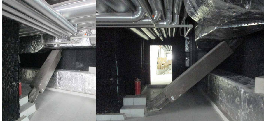
FIGURE 2.11 Example of the use of pipelines and service areas located at the outrigger storey (50-storey building in Izmir; photography by the author)
