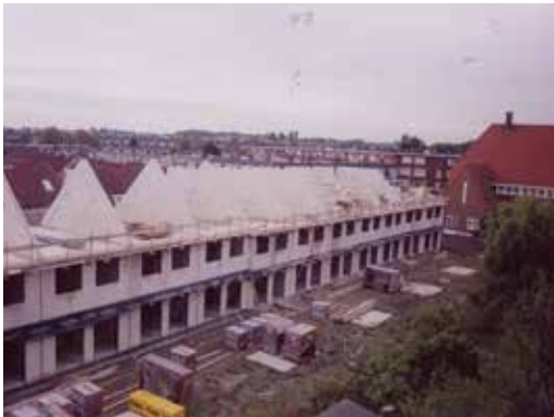
5 Construction in Tarwebuurt in the early 1980s
