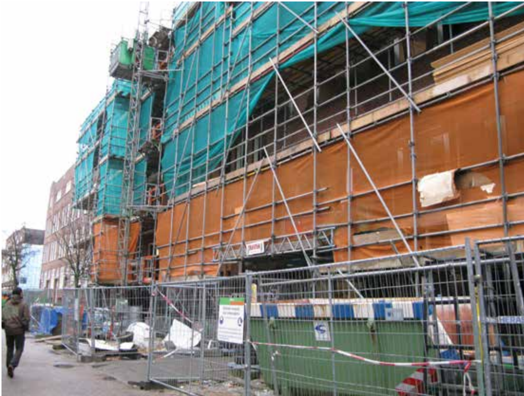
FIGURE 6.9 Housing renovation in Bas Jungeriusstraat in 2009
