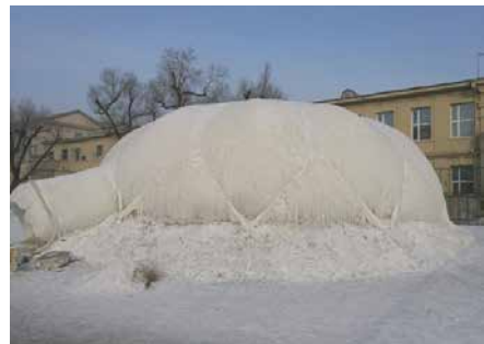
(b) Ice dome after construction.
