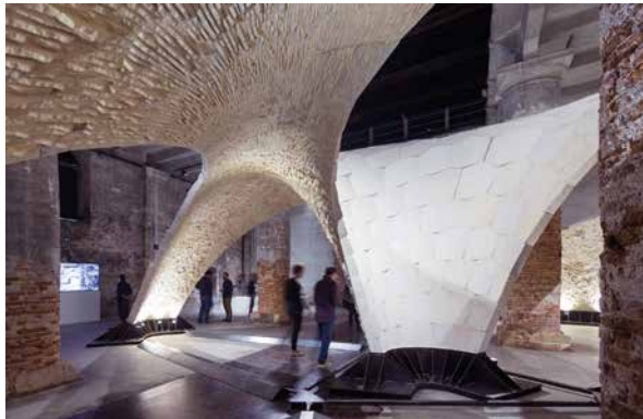
FIGURE 8.7 Tile vault prototype at ETH Zurich [151].
