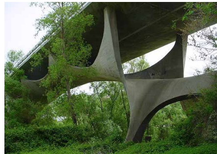
FIGURE 4.20 Figure 4.20: Basento Viaduct in Potenza, Italy, 1974 [108].
