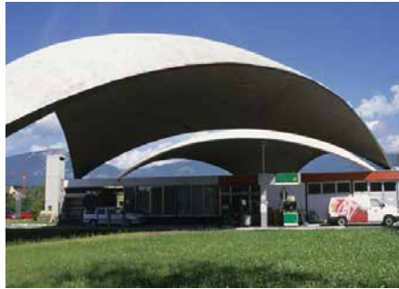
FIGURE 4.17 Deitingen Service Station, Switzerland, 1968 [104].
