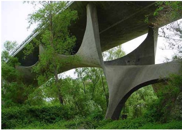
FIGURE 8.4 Supporting shell of the Basento Viaduct in Potenza [147].
