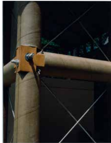
FIGURE 4.23 Photo of a wooden connector of paper tubes and post-stressed steel rods, 1991
