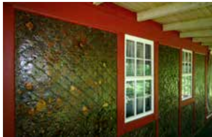
FIGURE 4.5 The Paper House in Rockport, Massachusetts, USA, outer wall 1924
