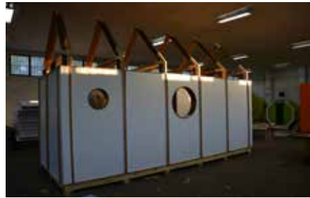
FIGURE 7.66 Construction of prototype- wall with large window
