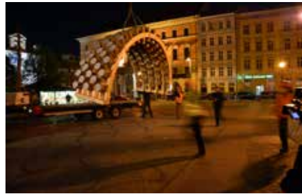
FIGURE 4.143 Placement the pavilion components on Solny Square, 2015
