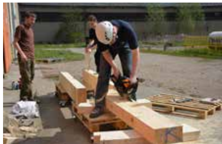
FIGURE 4.140 Preparing the wooden foundations, 2015
