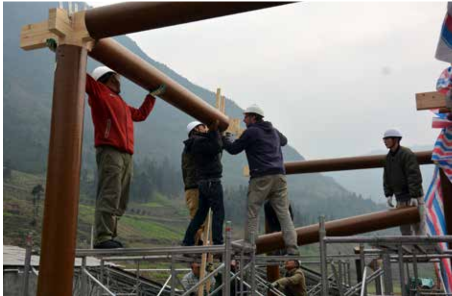
FIGURE 4.103 Miao Miao Paper Nursery School, construction of the paper tube structure, 2013
