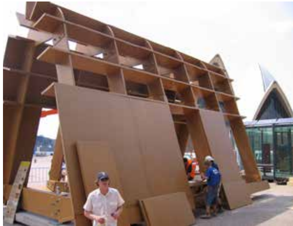
FIGURE 4.72 Cardboard House, Sydney, Australia, A-frame cardboard structure, 2004
