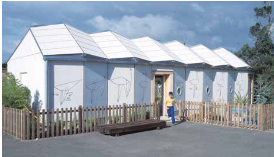
FIGURE 4.61 Westborough School, South façade, 2001
