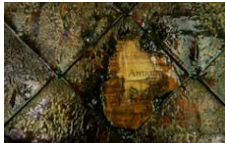
FIGURE 4.6 The Paper House in Rockport, Massachusetts, USA, 1924, detail of the wall
