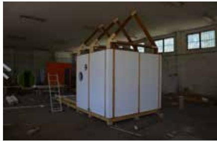
FIGURE 7.65 Construction of the prototype
