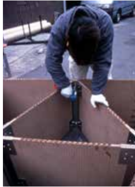
FIGURE 4.54 Nemunoki Children's Art Museum, construction of the roof, 1999
