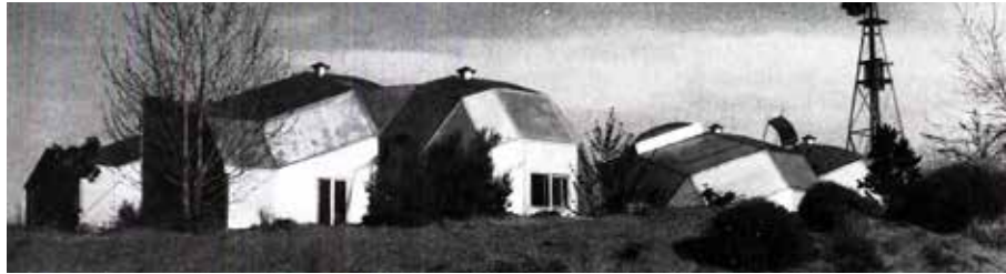
FIGURE 4.13 Baer Zome house, Corrales, New Mexico, 1971
