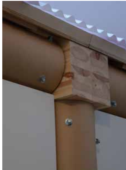
FIGURE 4.82 Hualin Primary School – 1:1 scale mock-up, timber joint detail, 2013
