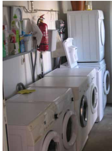
FIGURE 6.3 Launderette, Berlin (Germany) (picture: Tussen Ruimte 2012)
