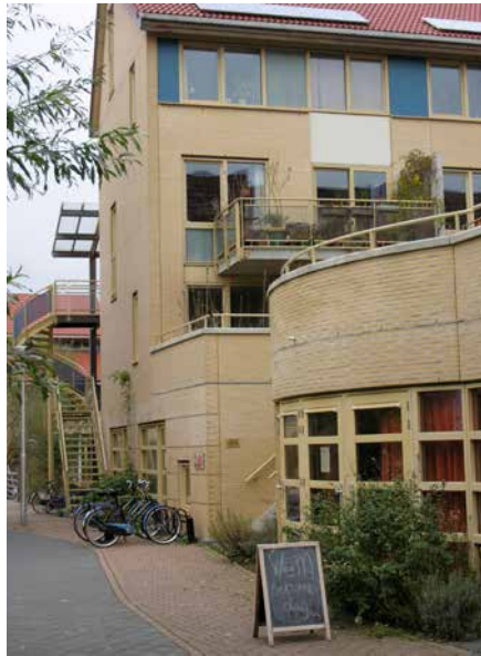
FIGURE 6.2 Common house and roofgarden, Utrecht (NL) picture: Tussen Ruimte 2012)
